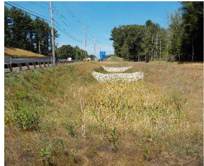
Vegetated Drainage Swale with Check Dams
